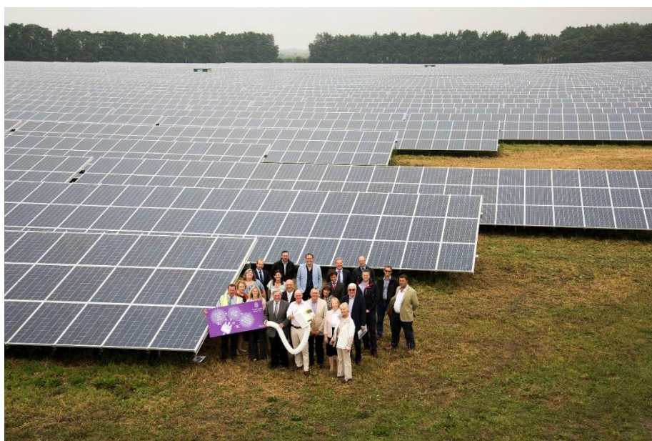
Toggam Farm – the largest Solar Farm in public ownership in the UK
